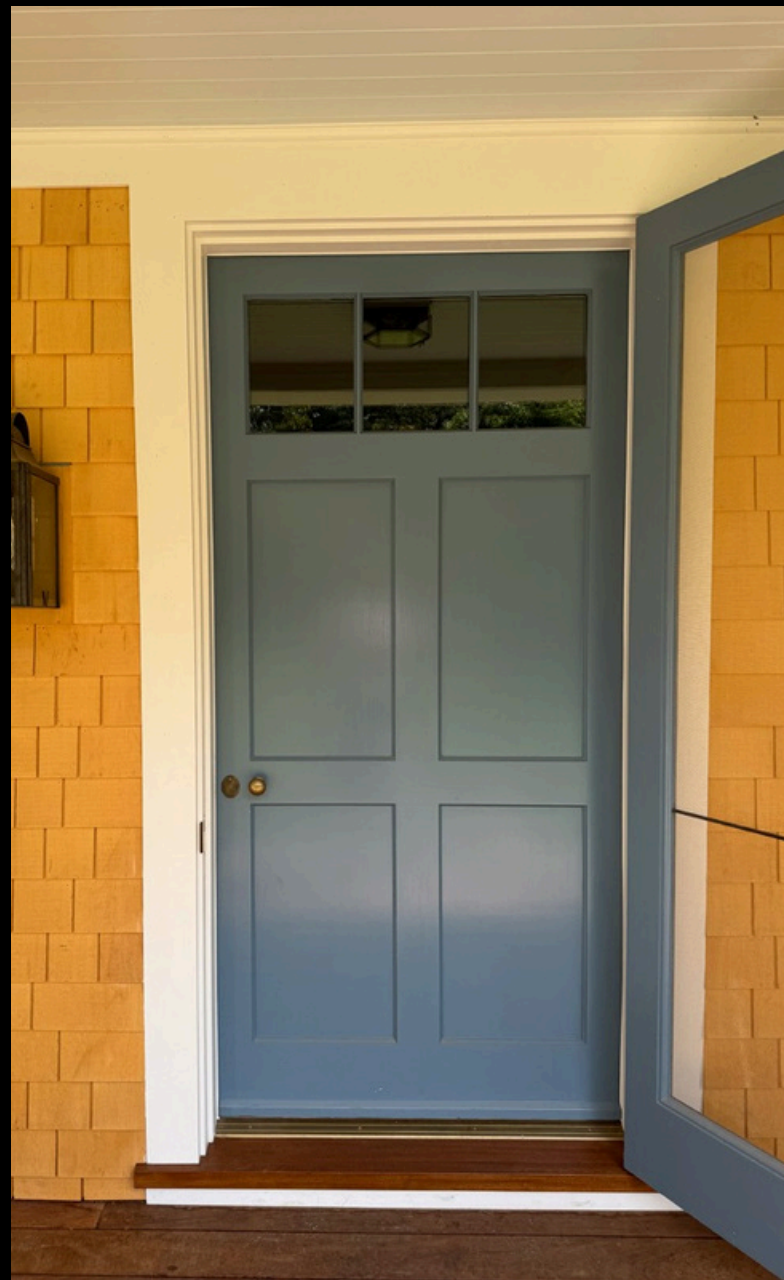
South Porch Entrance
