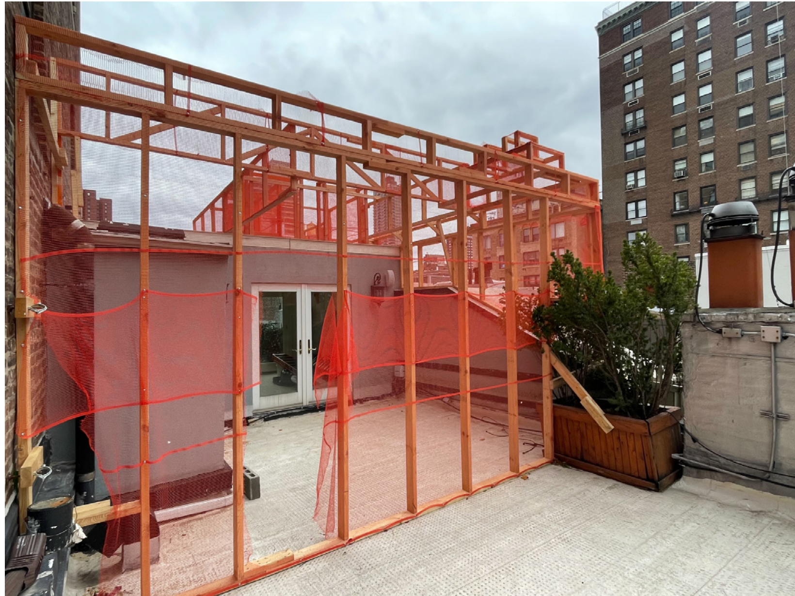
VIEW OF THE MOCK-UP FROM THE FRONT
