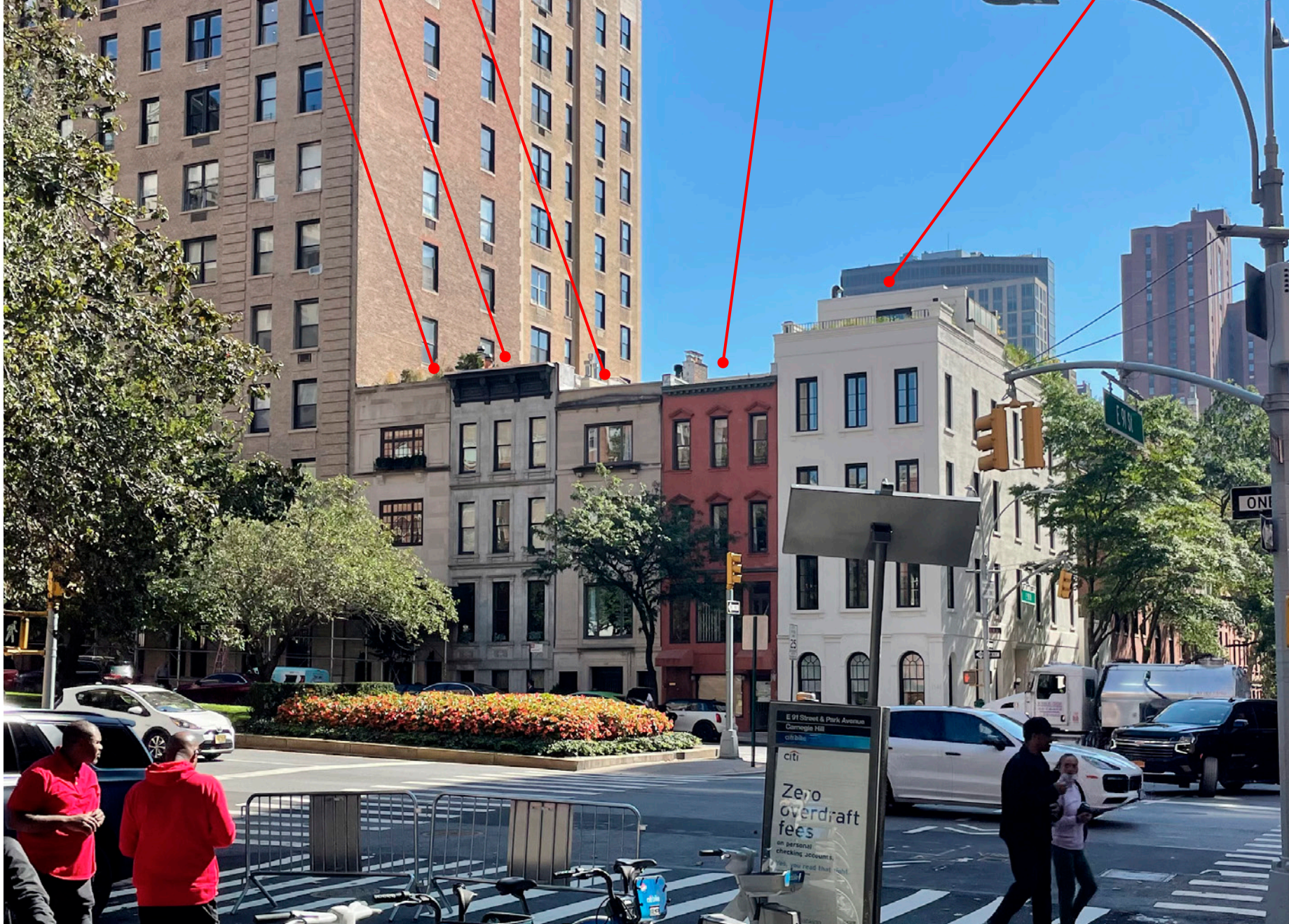
View of the east side of Park Avenue, between East 91st and 92nd Streets.
