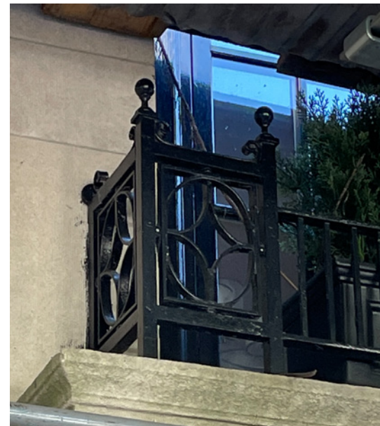
4. WROUGHT IRON RAILING
