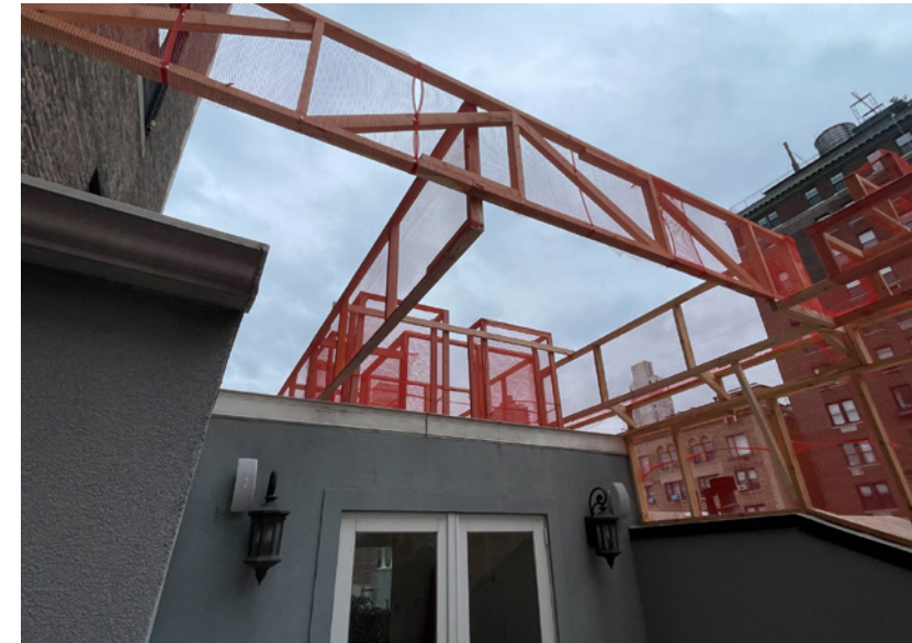
VIEW OF THE MOCK-UP FROM THE FRONT
