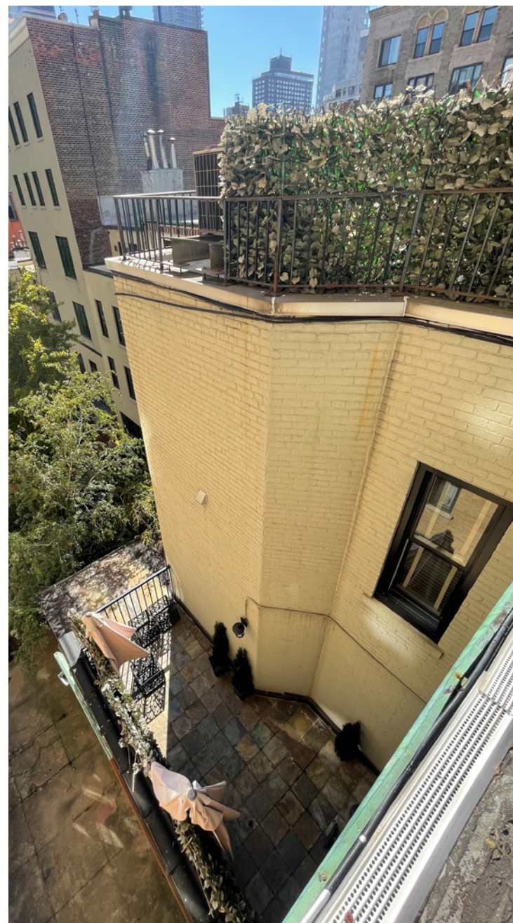
3. View looking down at the two-story rear extension.
