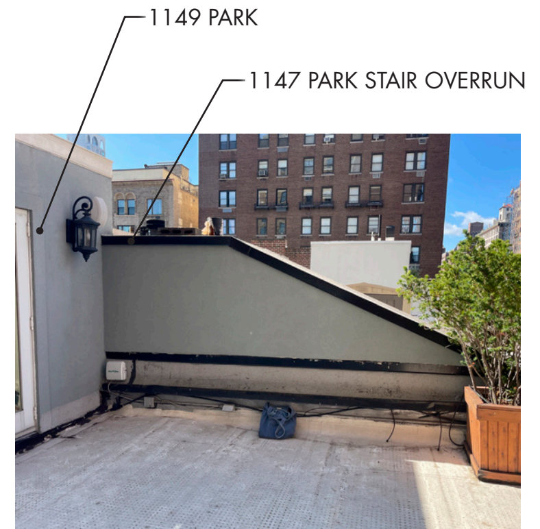
Rooftop view looking south towards the stair bulkhead at 1147 Park Ave.
