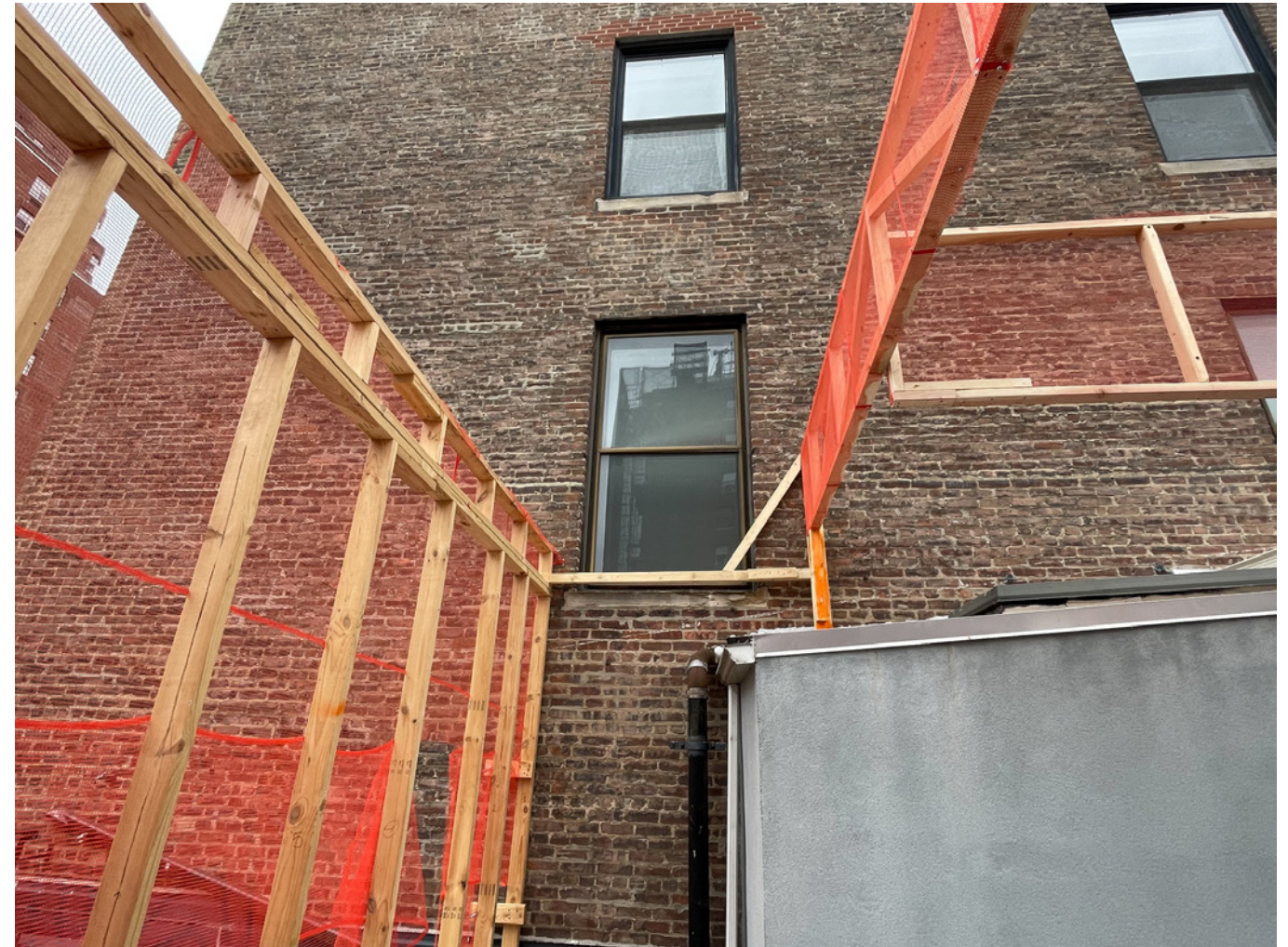
VIEW OF THE MOCK-UP FROM THE FRONT
