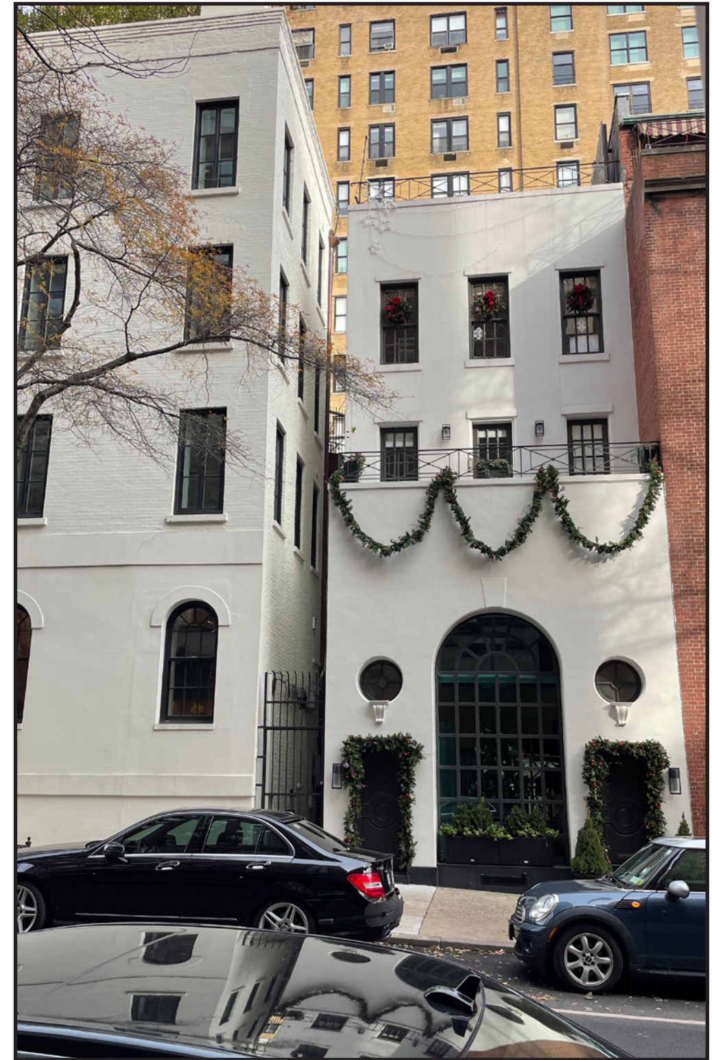
7. VIEW OF REAR FROM ALLEY ON 91ST STREET (NOT VISIBLE)
