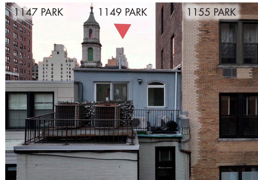
Rear view of the penthouse.
